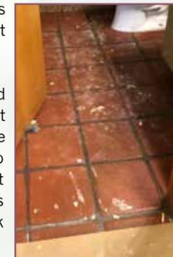
Once that was done, the paper was taken off of the floors again, so the concrete guy could come in and use self-leveling concrete over the whole large room.
