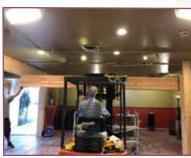
Here is then a picture of my dad using the forklift to lift up the beams to span where we took out the walls. The construction guys were really thankful to not have to lift up the beams themselves, like they normally have to! Once the beams were in, they put drywall up on some of the wall, and made the other walls a smooth surface. All of this was done with the floors
